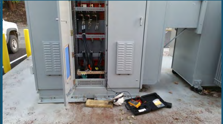
Fire Station Electrical Upgrade
